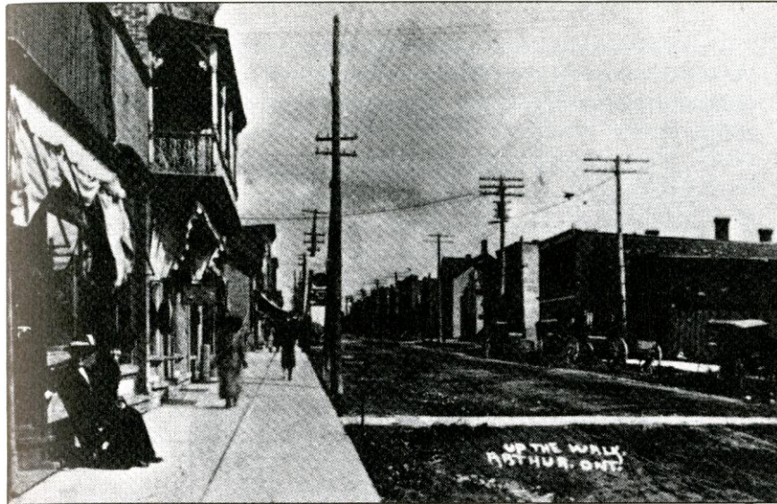
Promoting the Town with Cement Sidewalks: Arthur's boosters felt right up with the times with their new Main Street sidewalks in 1902.
