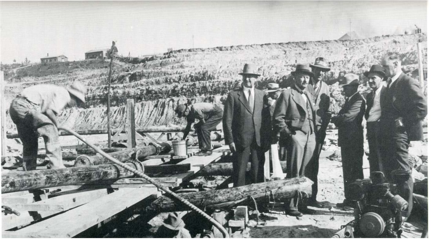
Grand River Conservation Commission at the Shand Dam, September 19, 1939. On the left, workmen disconnect and flush sections of the pipeline carrying concrete.
