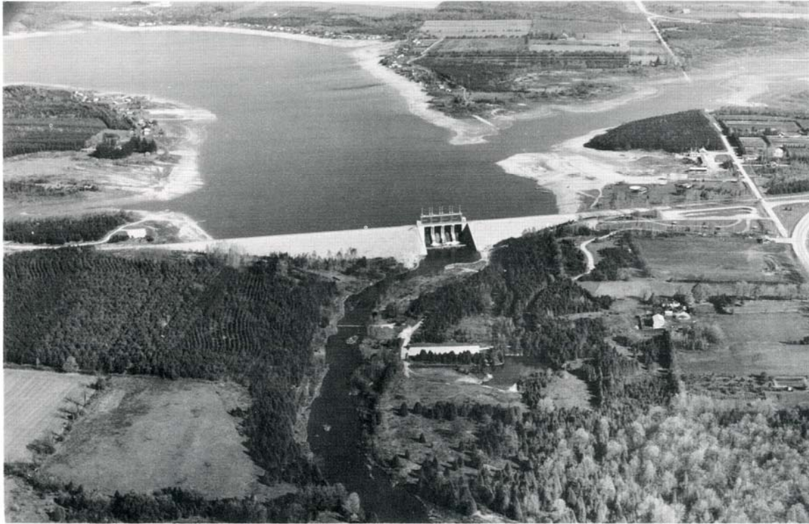
A modern aerial view of the Shand Dam, taken during the late summer when the lake level has been reduced to keep the Grand River flowing downstream.
