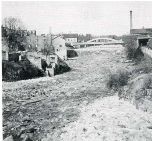
Six months later (February, 1937) record-breaking floods swept down the Grand. The dam is almost obscured by ice and water in this view. The water level is over 10 feet higher than the previous summer's, and it's moving fast!
