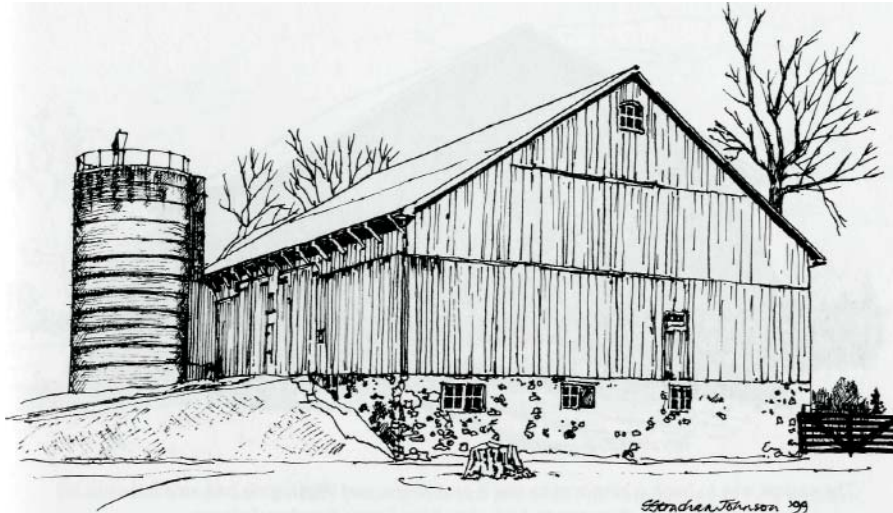
Raised barns were constructed at two levels - the ground stable and the second storey drive floor; pen and ink sketch by Susan Strachan Johnson.
