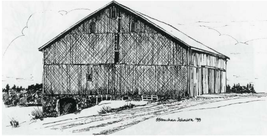
The easiest way to bank a barn was to site it on a slope, and Wellington had ample terrain for this; pen and ink sketch by Susan Strachan Johnson.
