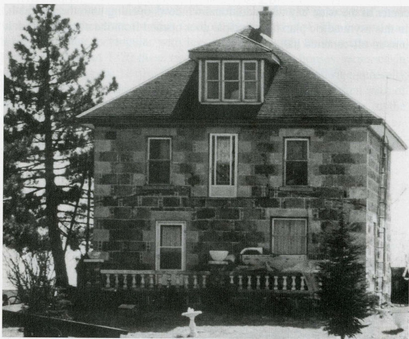
A cubic two-story farm house built toward the end of the nineteenth century using large blocks of field granite and limestone quoins. Lot 24 East, Concession 5, Eramosa Township.
