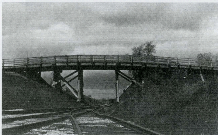
Canadian Pacific Railway bridge, Harriston, ca.1970; demolished 1976.
