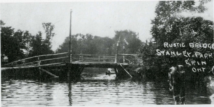
Rustic bridge, Stanley Park, Erin, ca.1910.
