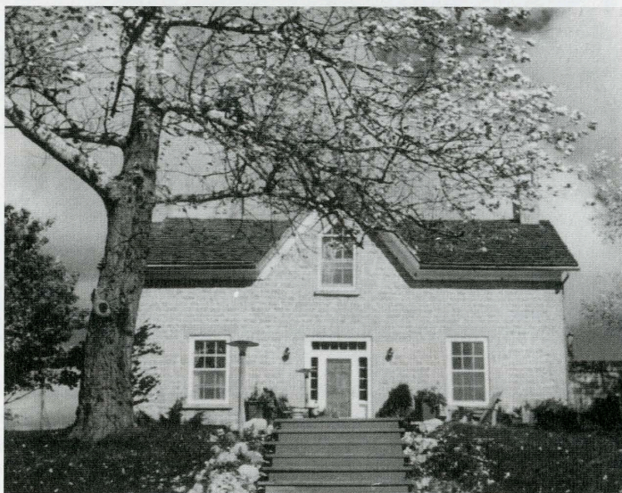
"Bon Accord" (1857) Lot 14, Concession 12, Nichol Township. The facade gable of this house, of coursed limestone, has a window with a triangular head. AUTHOR'S PHOTO. WELLINGTON COUNTY MUSEUM AND ARCHIVES, PH 15459.
