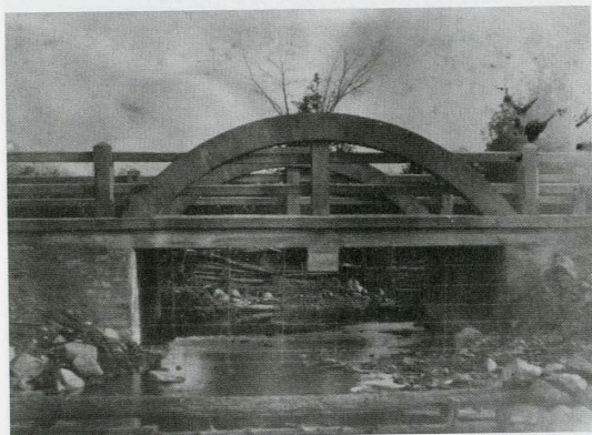
Concrete bridge, Clifford, ca.1920.
