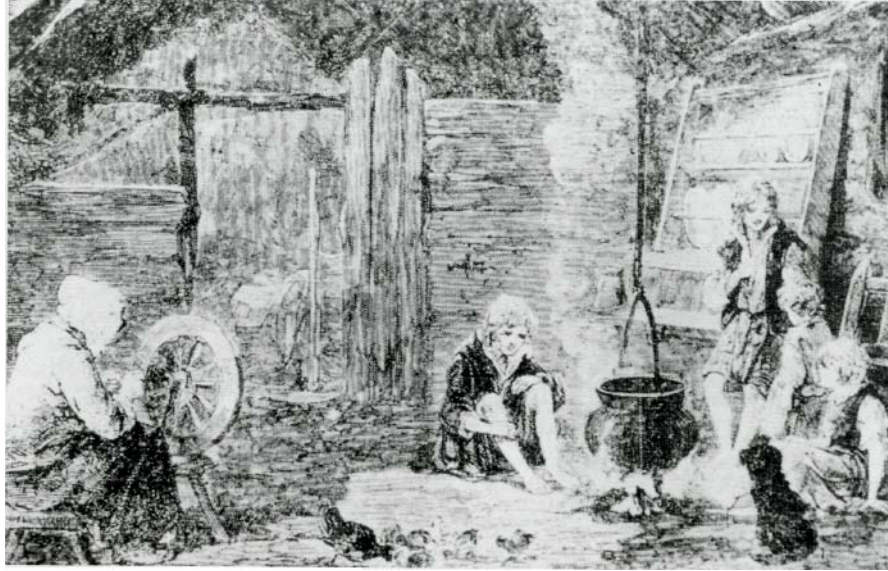
Figure 2: Interior of Skye cottage.
