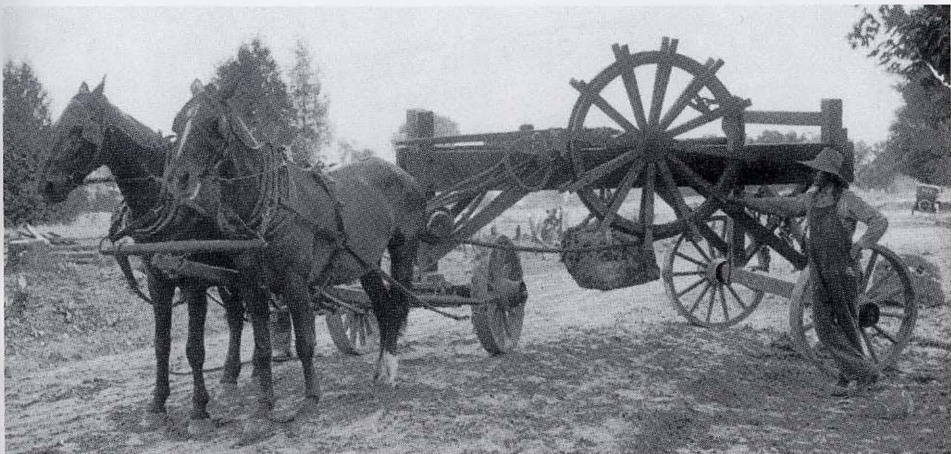
Boulder mover, used in road building, ca.1915.
